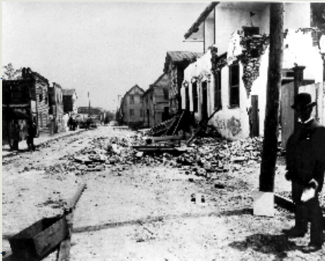
Charleston, South Carolina, Earthquake August 31, 1886. Fissure and a wrecked brick house on Tradd Street.
