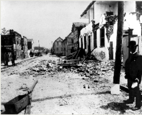
Charleston, South Carolina, Earthquake August 31, 1886. Fissure and a wrecked brick house on Tradd Street.
